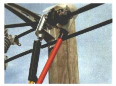
SHORT-CUTTING THE TWO STEP OPERATION WILL RESULT IN DAMAGE TO THE TOOL. THE MID-SPAN PART OF THE BLADE IS NOT DESIGNED FOR 25 & 35 KV INSULATION REMOVAL N ONE STEP.
