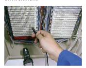
This locating method requires the use of a test tip which is part of a standard set.
