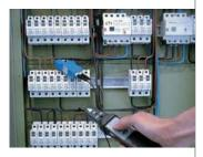
This tracing method uses A1074 current clamps.
